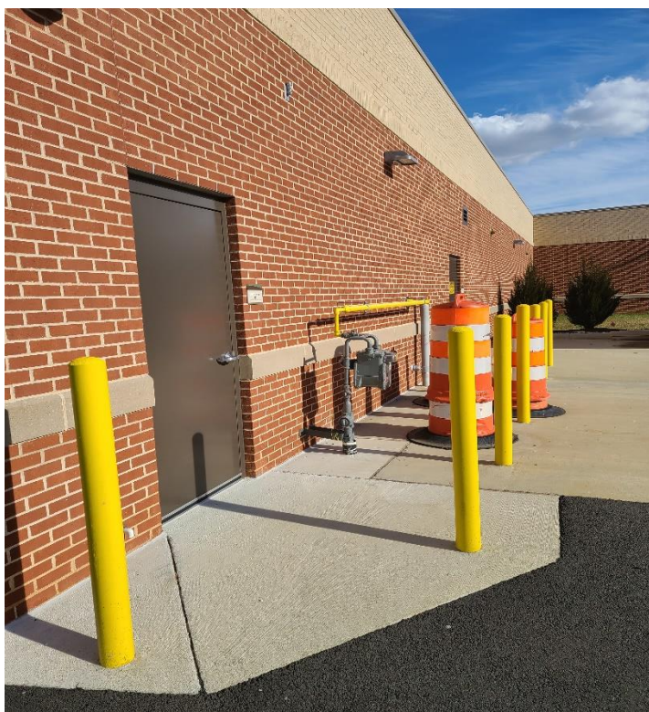
Gas meter base and shut off, exterior side Charlie
